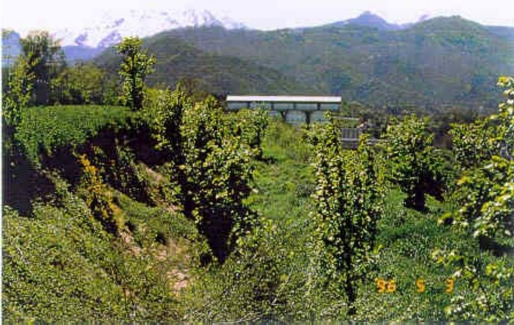
*Fig. 1 - The waste (right, under the surface of a closed landfill) settling along a steep slope of natural soil (left in the photo) may cause cracks in the peripheral portions of the waste body. An insufficient gas extraction system causes biogas to flow through those fissures. Biogas presence is revealed by the barren patches that are clearly visible in the vegetation of the final cover, and can be detected on-site with a simple, portable gas detector.*
